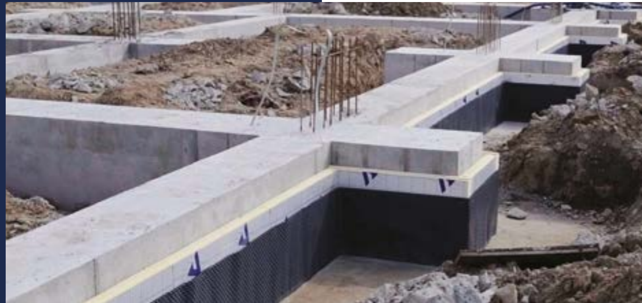
Insulation of foundations with termPIR® boards
