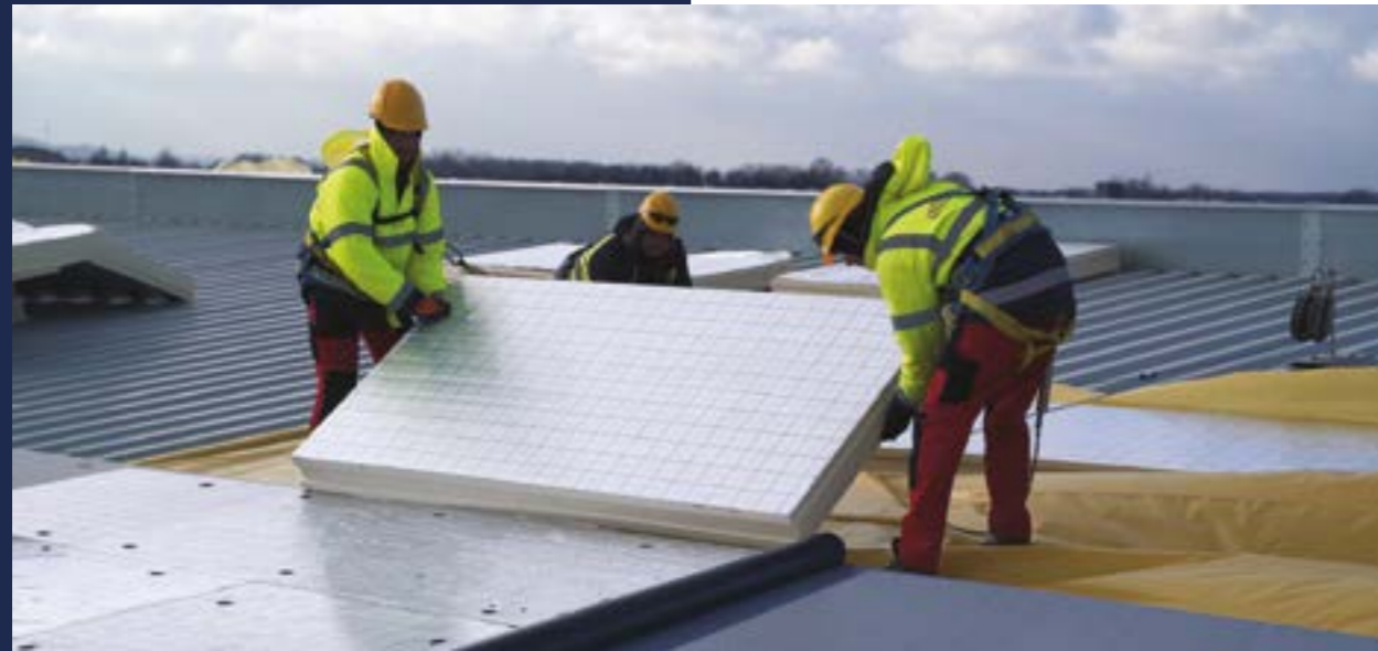
Installation of termPIR® boards on a flat roof
