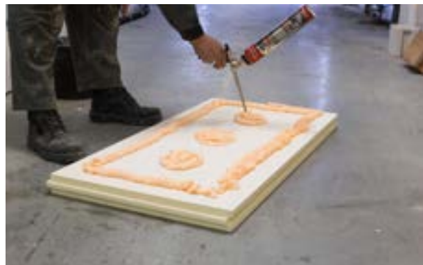
Photo 08. Distribution of polyurethane adhesive on the board.
