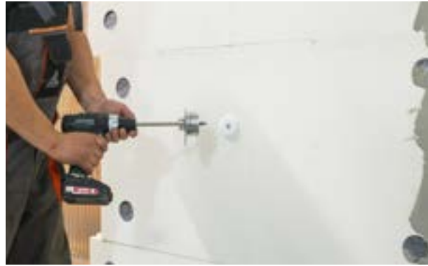
Stage IV c) Driving an anchor screw into an insulation layer.
