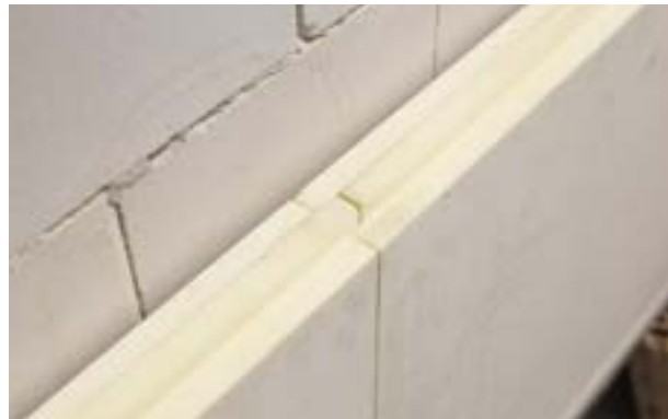
Photo 07. View of a properly positioned interlocking joint.
