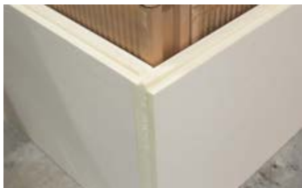
Photo 11. View of corner boards after installation.
