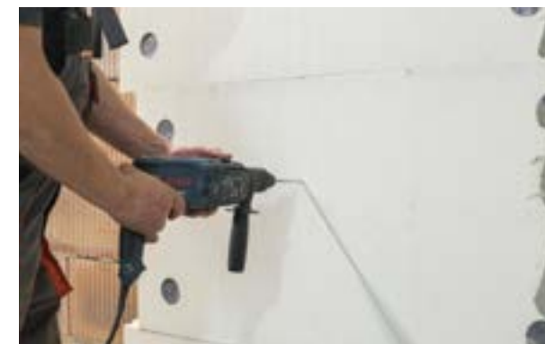
Stage IV a) Drilling a hole in the wall for an anchor screw sleeve.
