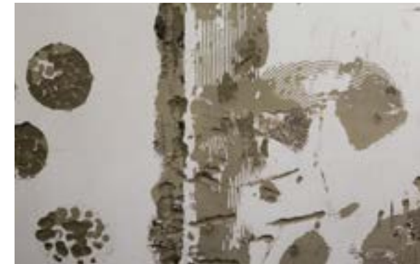
Photo 01. Cavities to be filled with adhesive.
