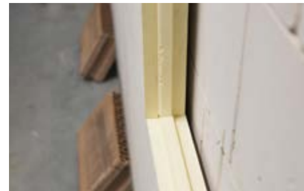
Photo 09. View of properly a positioned interlocking joint.
