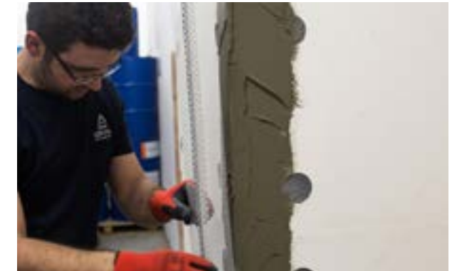
Stage V c) Installation of a pre-made corner.
