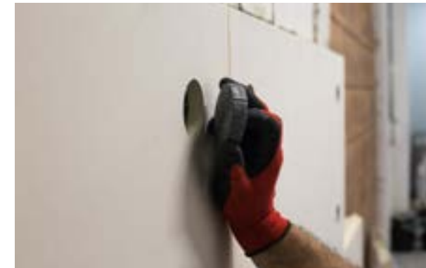
Stage IV e) Installing a cap.
