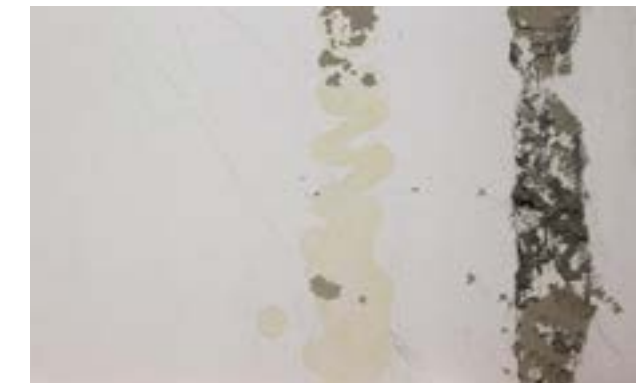
Photo 04. Spots that may reduce adhesion of the adhesive.
