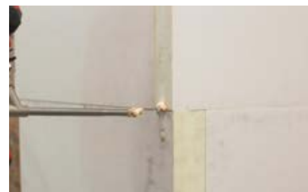
f) Filling roof outlets with low pressure polyurethane foam.
