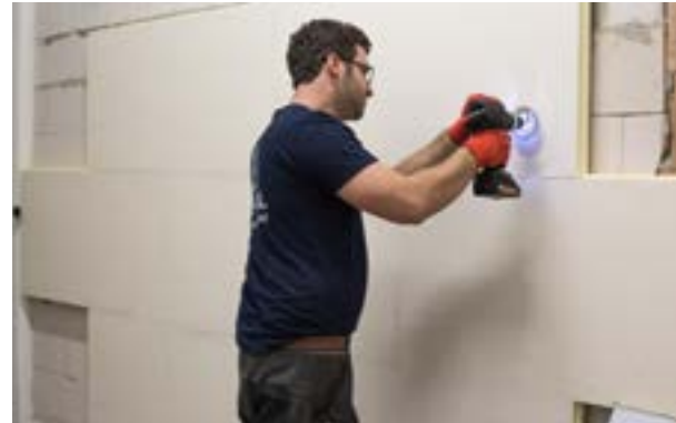
STAGE IV b) Making an opening in a board for an anchor screw sleeve.
