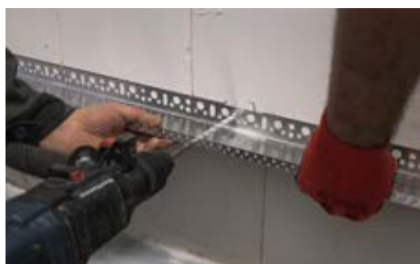
Stage I. b) Positioning and installing a starter strip.
