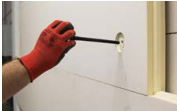
Stage IV c) Installing an anchor screw sleeve.
