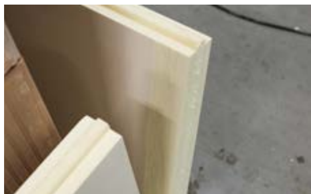
c) Installing corner boards.
