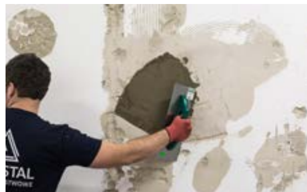
Stage III. Making a levelling layer on a previously prepared substrate.
