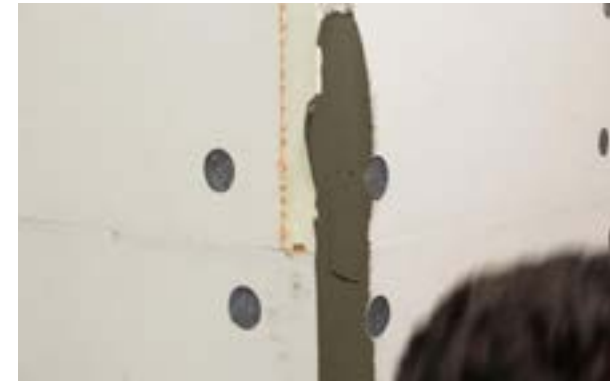
Stage V b) Applying a layer of adhesive in a corner.
