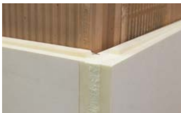
Photo 12. View of boards prepared for the installation of the next row.
