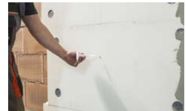
Stage IV b) Embedding an anchor screw.
