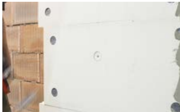
Photo 16. View of an anchor screw after installation.
