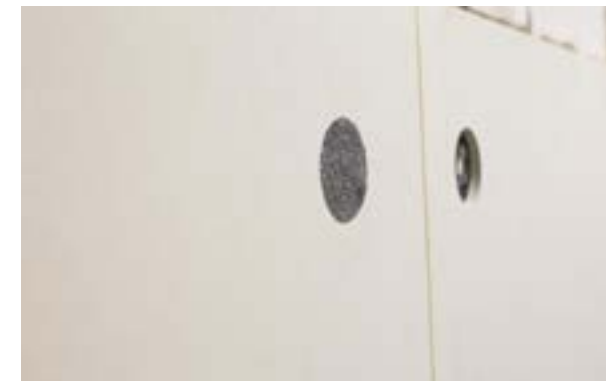
Photo 15. View of a cap after installation.
