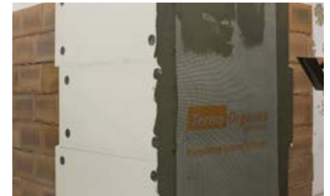
Stage V e) Installing reinforcing mesh.
