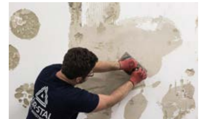
Stage I. Mechanically removing old plasters and adhesives as well as peeling paint.
