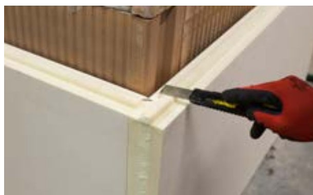
d) Removing the tongue of a corner board.
