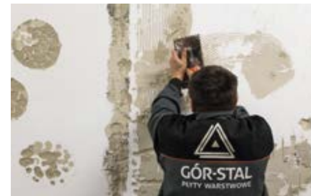
Stage I. Mechanically removing old plasters and adhesives as well as peeling paint.
