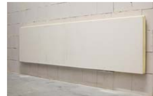
Photo 06. View of boards in place.
