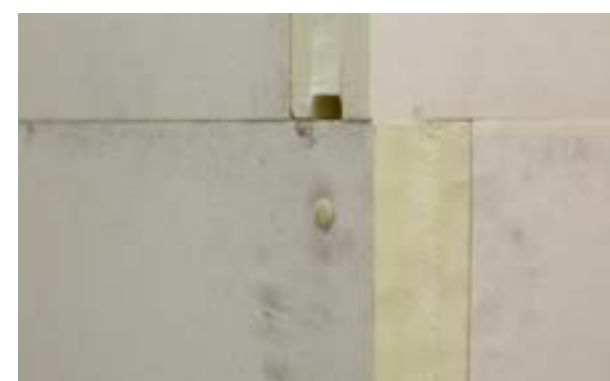
Photo 13. View of a component protecting a corner after installation.
