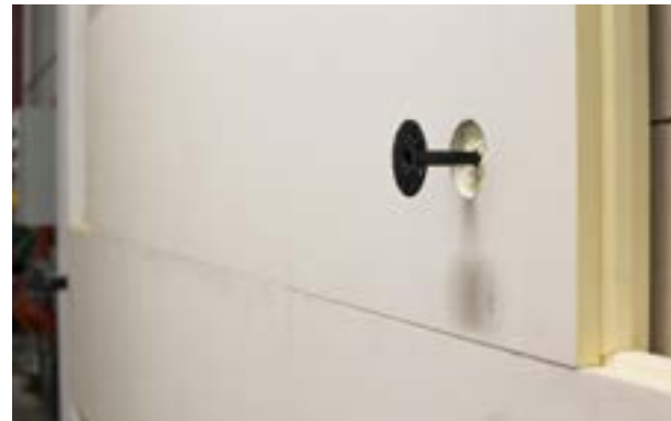
STAGE IV b) Making an opening in a board for an anchor screw sleeve.
