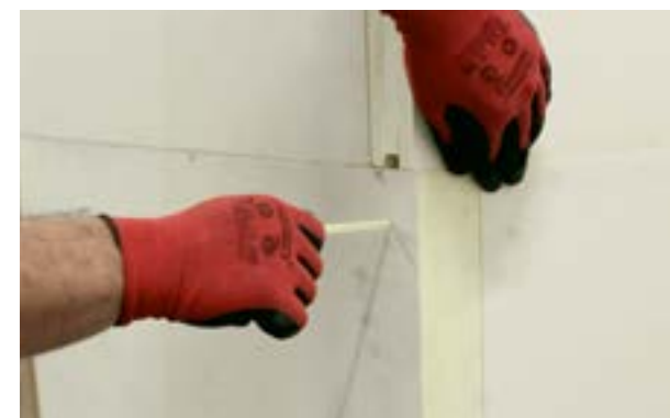
e) Installing plastic connectors preventing corners against deformation.
