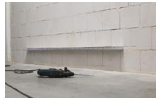
Photo 05. A properly installed starter strip.
