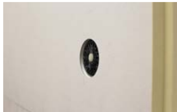
Photo 14. View of an anchor screw after installation.
