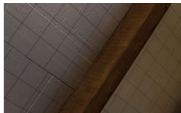
Photo 05. Roof view from inside without full boarding This requires finishing with, for example, dry plaster.
